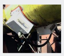
MoistScan® MA-600 installed on a large screwfeeder conveying woodchips to a dryer at a wood char plant. Data from the MoistScan® is used to control the dryer such that the woodchip exiting the dryer is between 5-12% moisture.
