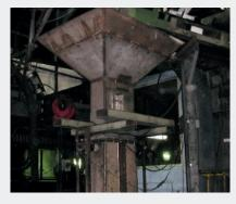
MoistScan® MA-600 installed on the wall of a hopper feeding a briquetting press at a briquetting factory. The material is a mixture of sand, sodium nitrate and char. Control of the moisture content of the briquettes is critical. If the mixture is too dry the briquettes don't form correctly. If the mixture is too wet the briquettes may split in the fluidised bed dryer or in transit.
