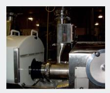
MoistScan® MA-700 analyser installed on the in-feed to a hydrator at a snack foods factory. The analyser measures the moisture in a mixture of polenta and rice. Data from the MoistScan® directly controls moisture addition to the hydrator to ensure the product meets quality specification.
