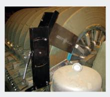
MoistScan® MA-600 installed on a vertical disk filter at a copper processing plant. The analyser measures the moisture in filter cake Data from the MoistScan® controls the vacuum pressure of the filter plates to produce a filter cake within a tight moisture specification of 7-8%.
